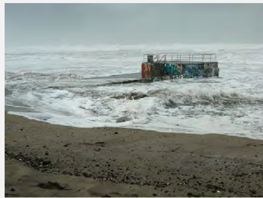
Discharge of Treated Wastewater
