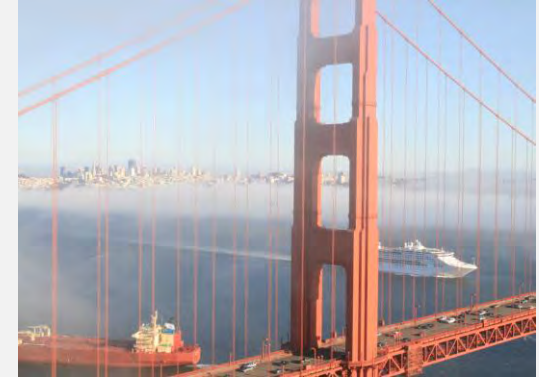
Presence & Level of Vessel Traffic
