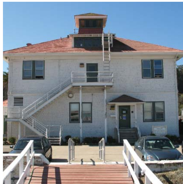
Fig. 38 :North elevation, the current window configuration of the Life Safety Station.
