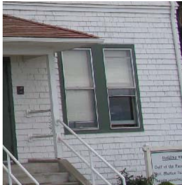
Fig. 54: Double-hung window at the Main Boathouse
