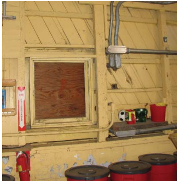
Fig. 62 : Diagonal board walls at the Shop & Garage.
