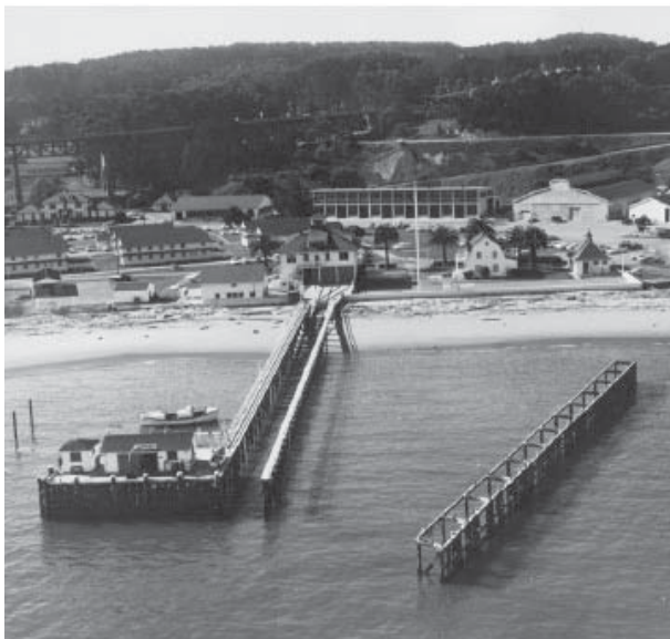
Fig. 10: Boat launch and pier with Buoy Shack and Tide Gauge House, 1958.
