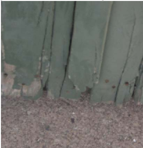
Fig. 45: Mechanical deterioration of doors of the Shop & Garage associated with cross-grain dragging.
