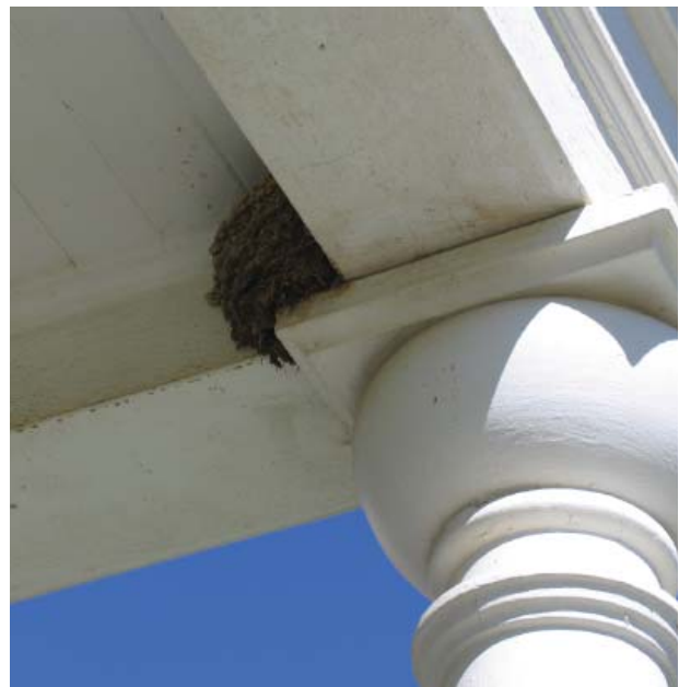
Fig. 30 : Mud Swallows nesting in the eaves of the porch at the Officer in Charge Quarters.
