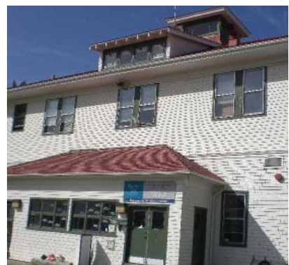
Fig. 23 : East elevation of the Main Boathouse.
