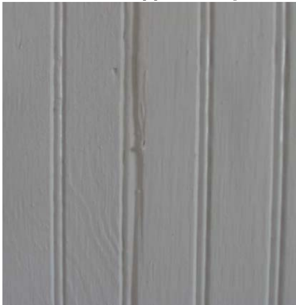
Fig. 61 : Beadboard wall cladding in the Buoy Shack.
