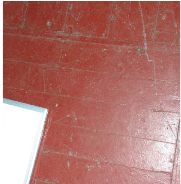
Fig. 66 : Original wood flooring at the Shop & Garage.
