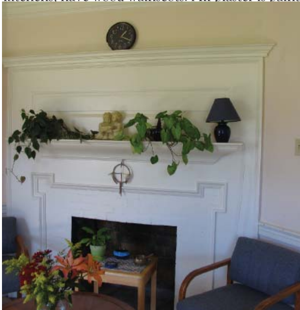
Fig. 63 :Painted wood fireplace, mantle, and wooden elements at the Officer in Charge Quarters.
