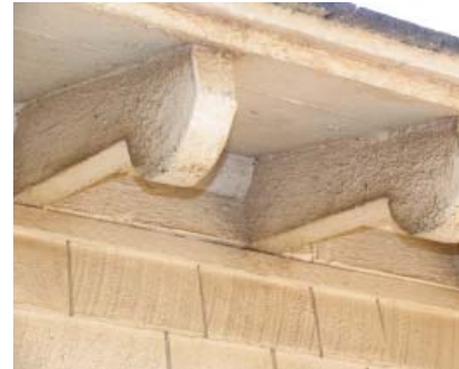
Fig. 14 : Detail of Rounded Exposed Rafter Tails.
