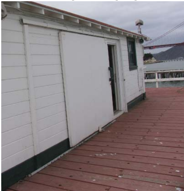
Fig. 47: Sliding wooden door at the Buoy Shack
