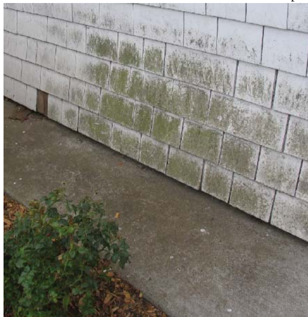
Fig. 35 : Biological growth has developed in moist, shaded areas
