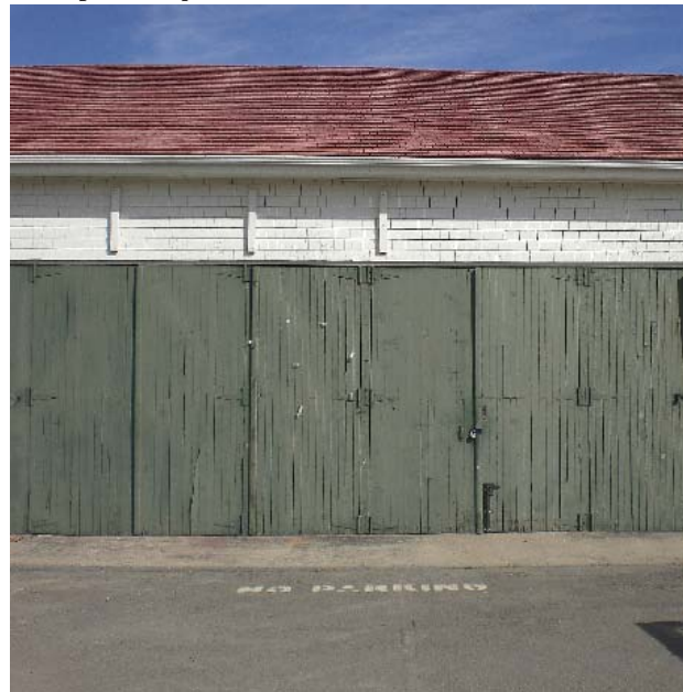
Fig. 48: Vertical tongue-and-groove wood doors at the Shop & Garage.
