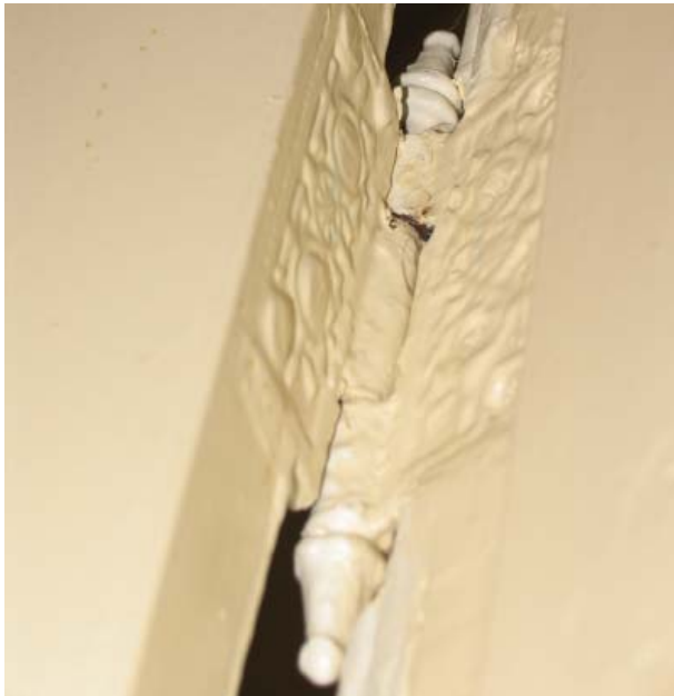
Fig. 69 : Original hardware at the Officer in Charge Quarters.
